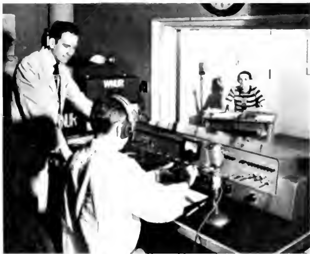
CONTROL ROOM IN BROADCASTING STUDIO
